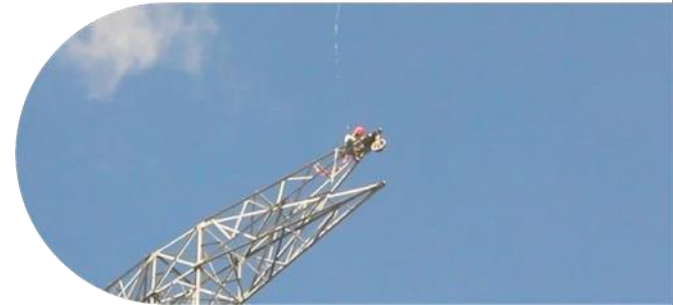
Laying of nylon thread
