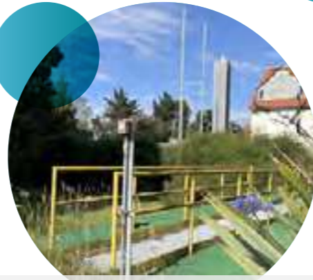
Gas Compression Station La Sabana
